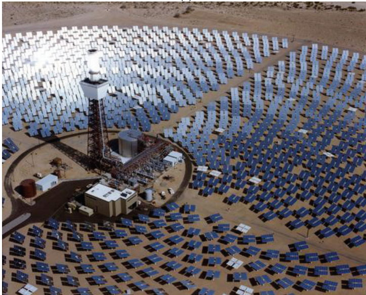
Fig. 21. (a) Schematic of a power tower. Image adapted from Energy Efficiency Renewable Energy Network {J. Tidwell, 2005} [61]; (b): Solar Two, power tower. Image courtesy of NREL's Photographic Information Exchange [62].
